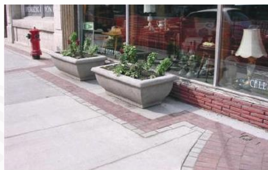
Figure 81: Contrast Border Texture and color-contrast border at obstacle.
