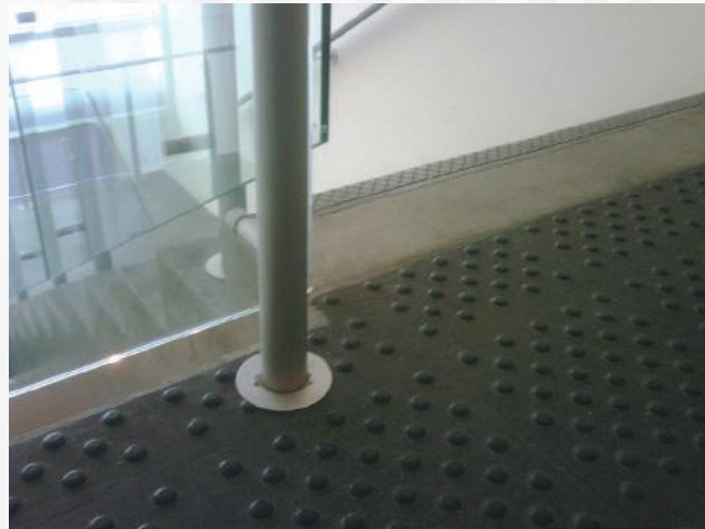
Figure 216: Detectable Warning Surface at Top of Stair
