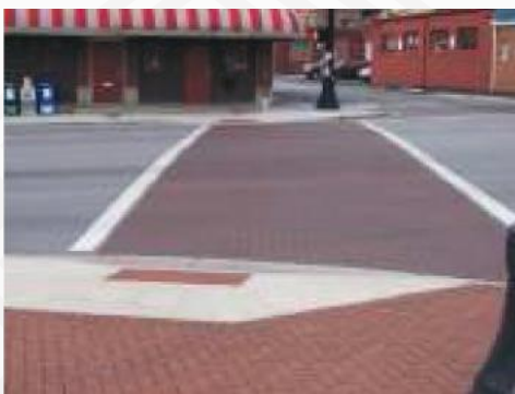
Figure 56: Detectable Warning Surfaces
