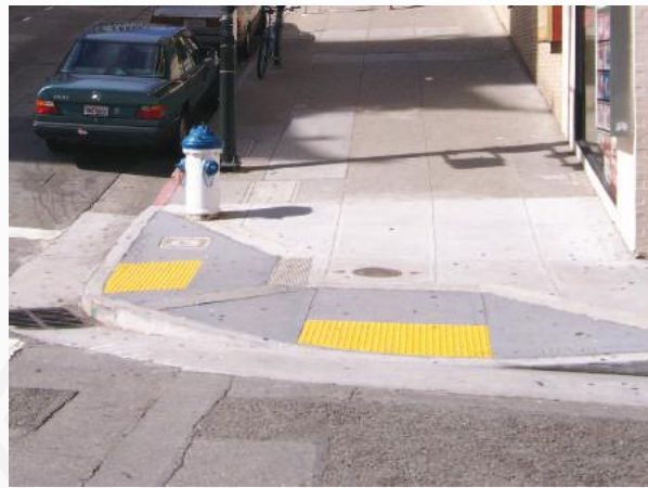
Figure 215: Detectable Warning Surface at Kerb cut
